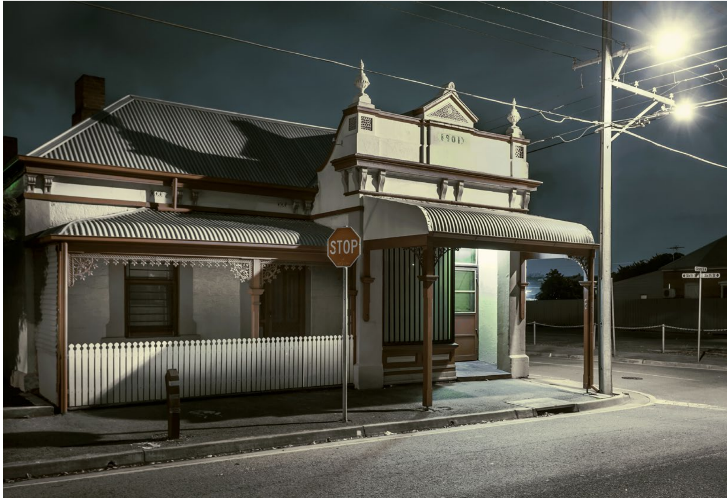
'1901' historic former shopfront at night. Bowden, Adelaide, Australia. Canon EOS 5D MkII with 17-40mm f4 L lens. © Wayne Grivell
